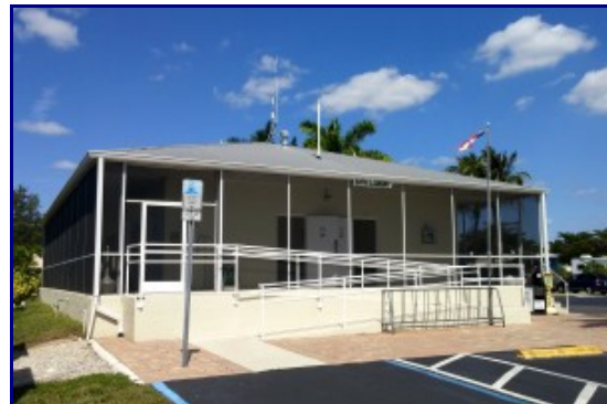
The bath/laundry building
