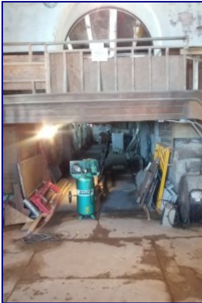
Bowling alleys (in progress)
