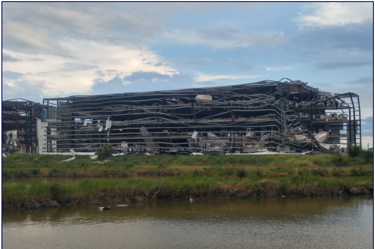
Wrecked 5-story boat storage facility
