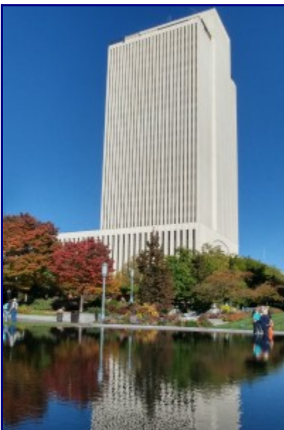
LDS office building
