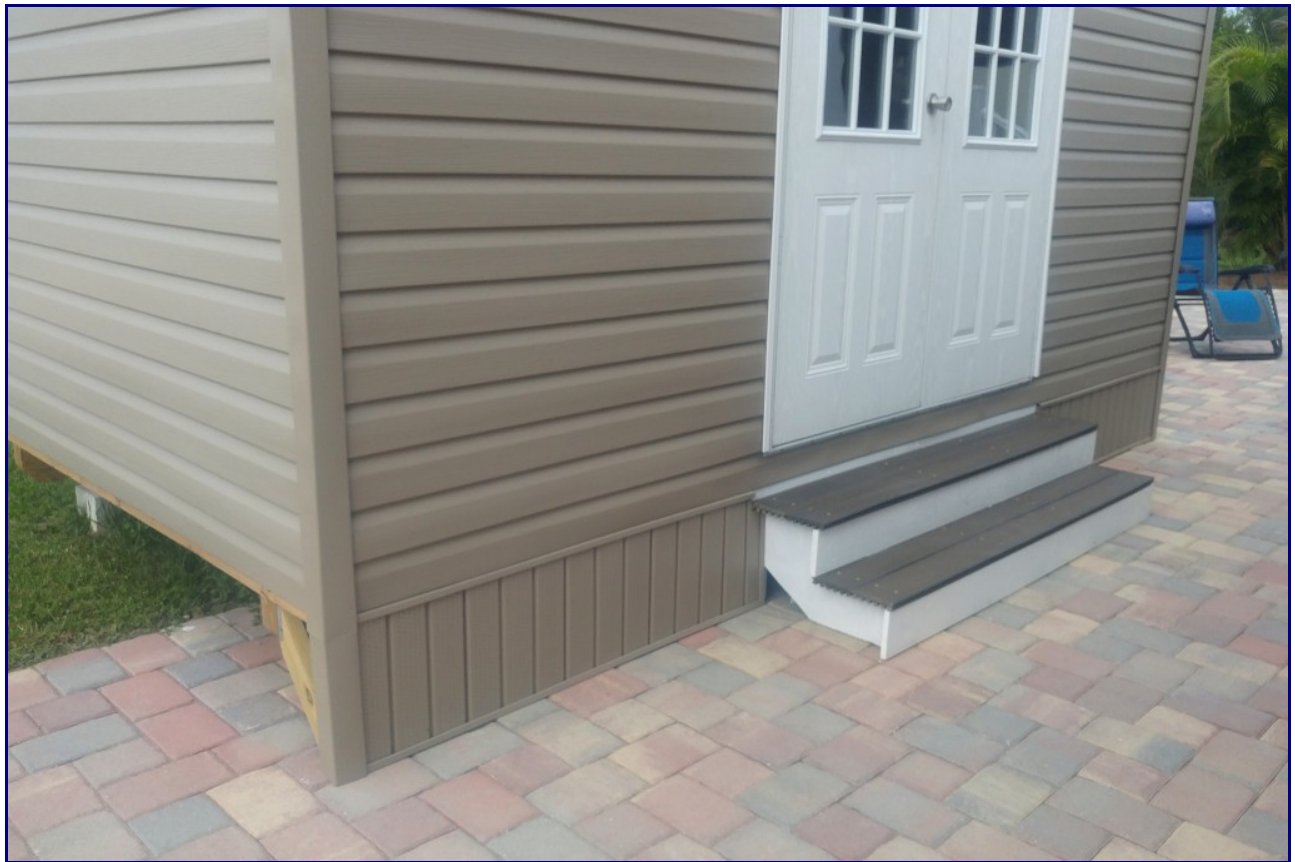
Skirt on the front of the shed
