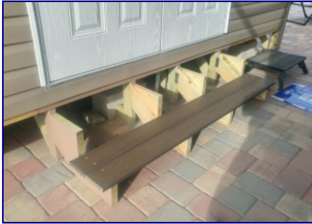
Construction getting started
