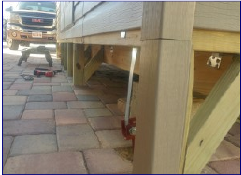
The shed frame
