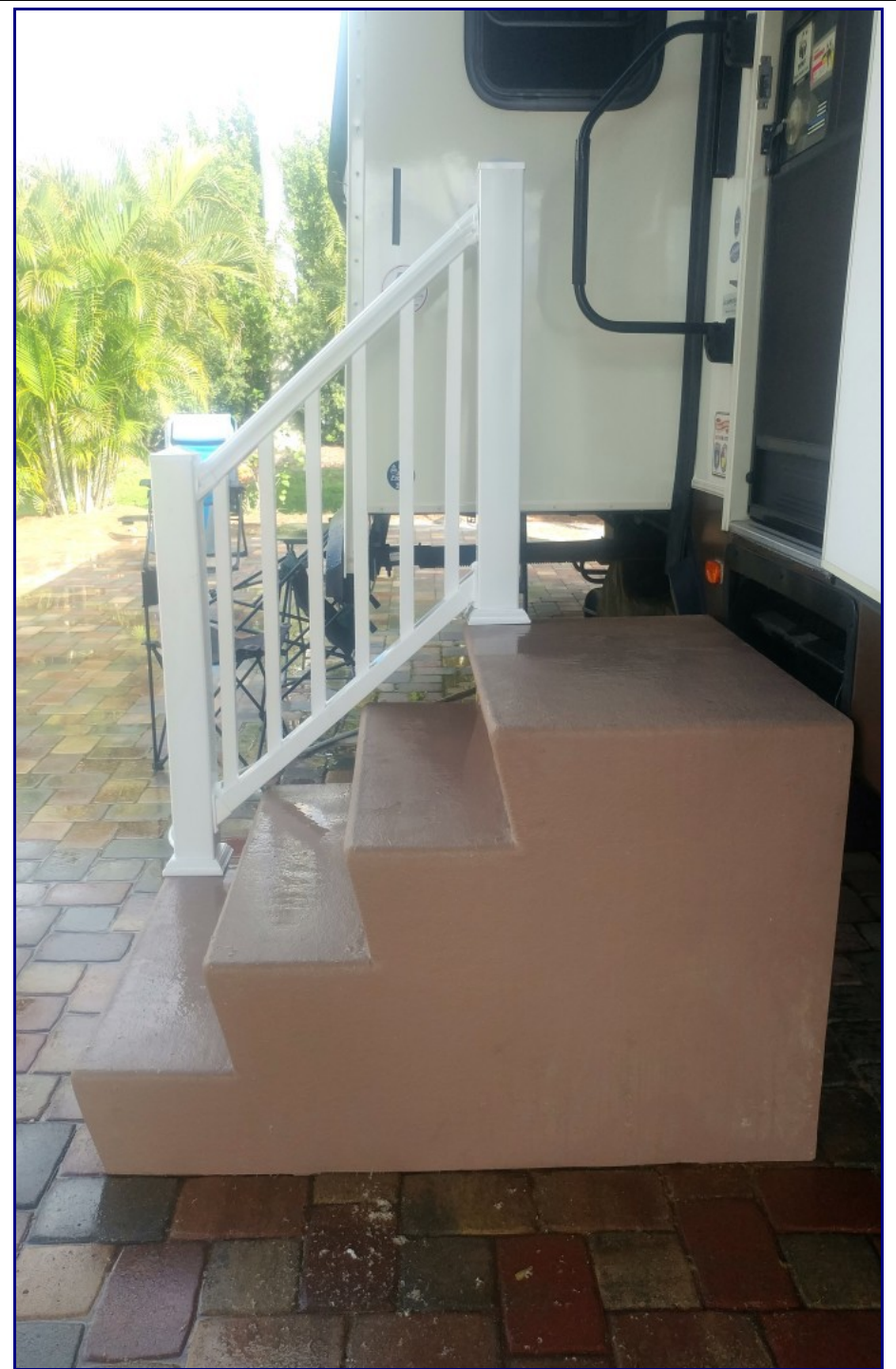
The finished railing on painted steps
