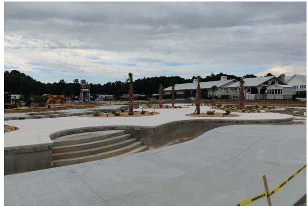
Water park in progress
