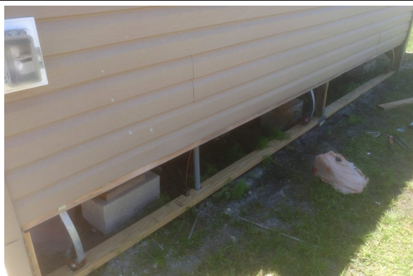
Framing the side
