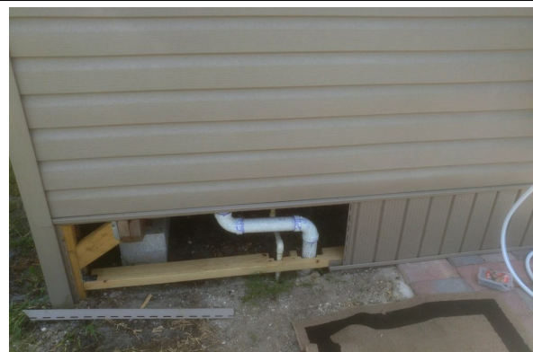
Framing the front
