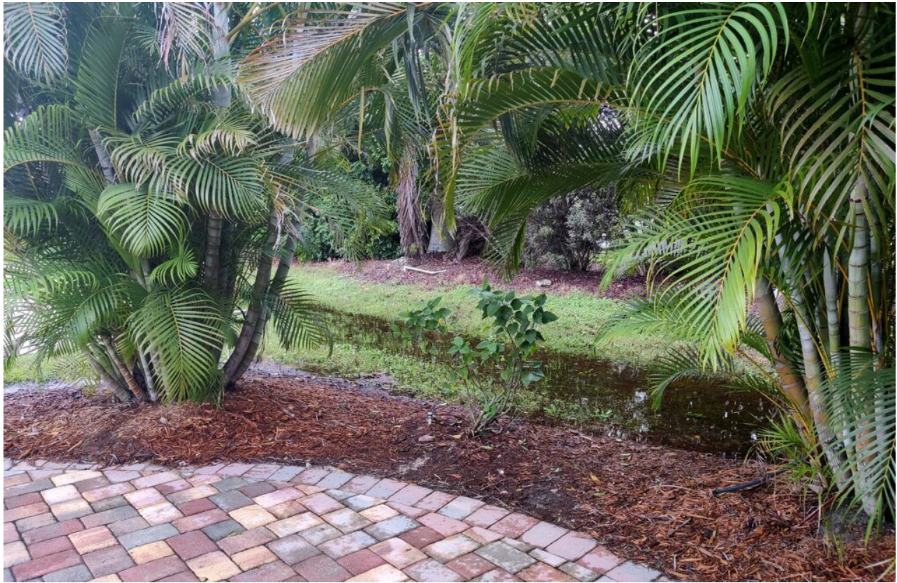
Flooded drainage ditch, second pass
